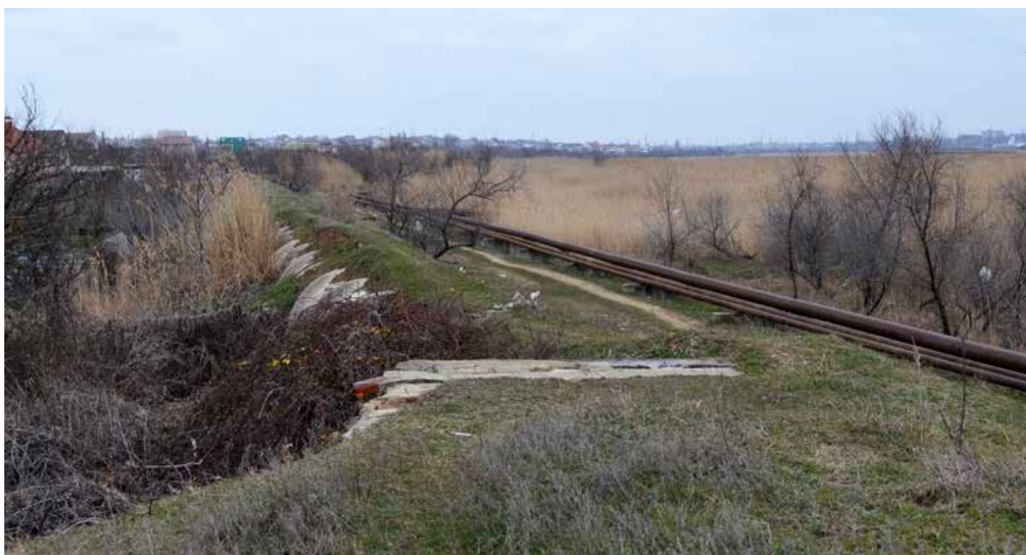
A culvert and a mothballed pipeline near Zymivnyk, Kherson.
